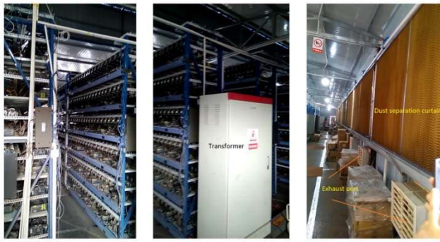
Figure B. A GPU mining farm in China Source: NVIDIA Corp.
